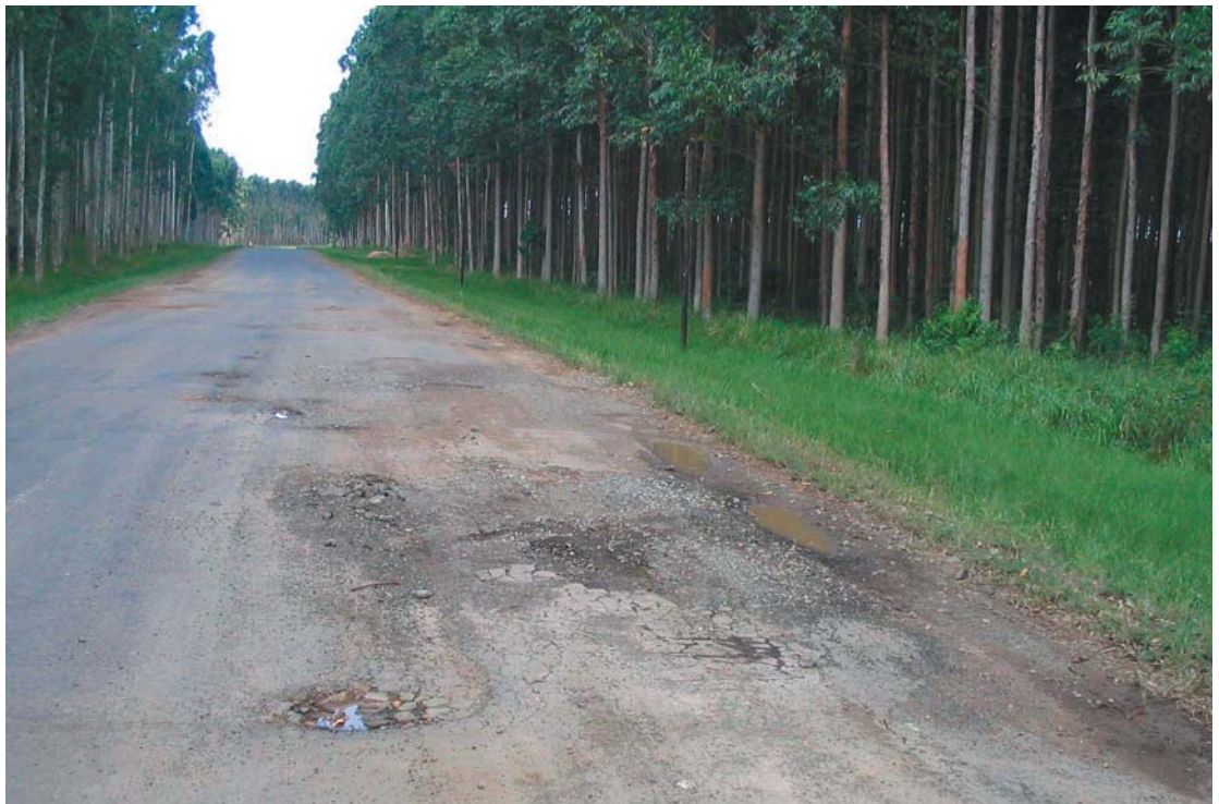
Roads near Mavuya are damaged by heavy timber trucks creating dangerous conditions for other motorists
