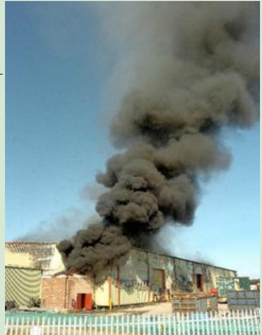
Photograph 11: Fire at Scotgen's Dargavel plant
