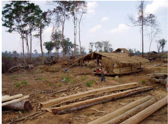
Village lands being cleared for Oji Paper's industrial tree plantations, Pakkading, Bolikhamsay province, March, 2006.
