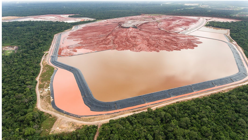
Barcarena, Brazil, tailings dam. Ph: Pedrosa Neto
